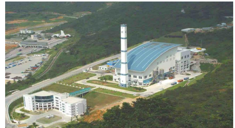
Waste to energy station
